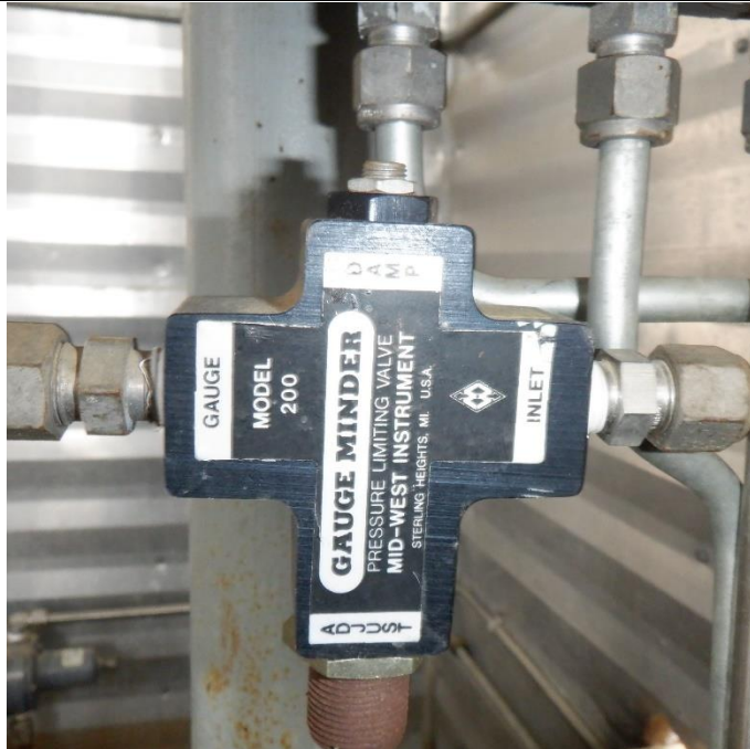
Pressure limiting valve overview.
