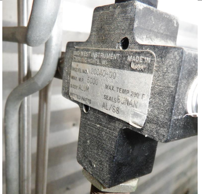
Pressure limiting valve overview.
