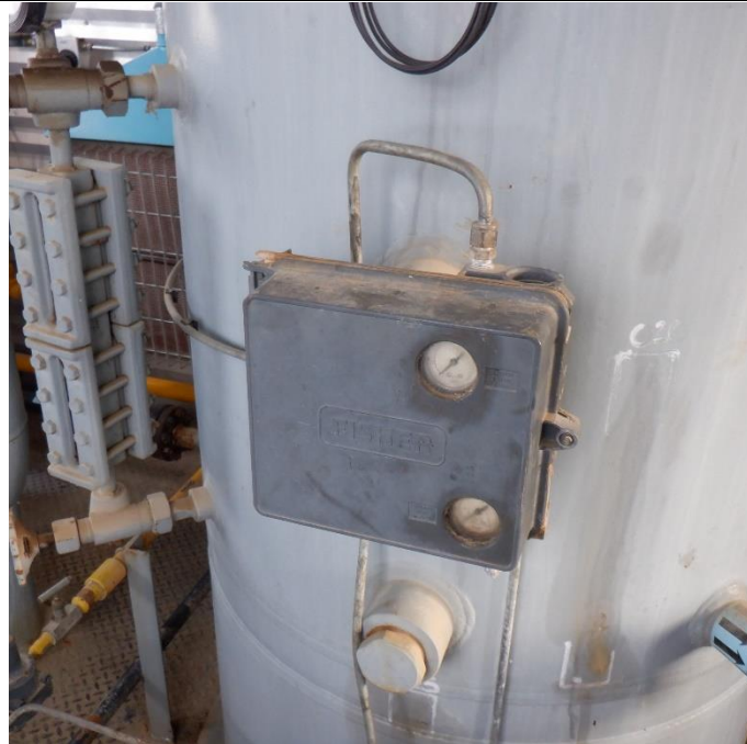
L/O level controller sealed shut.
