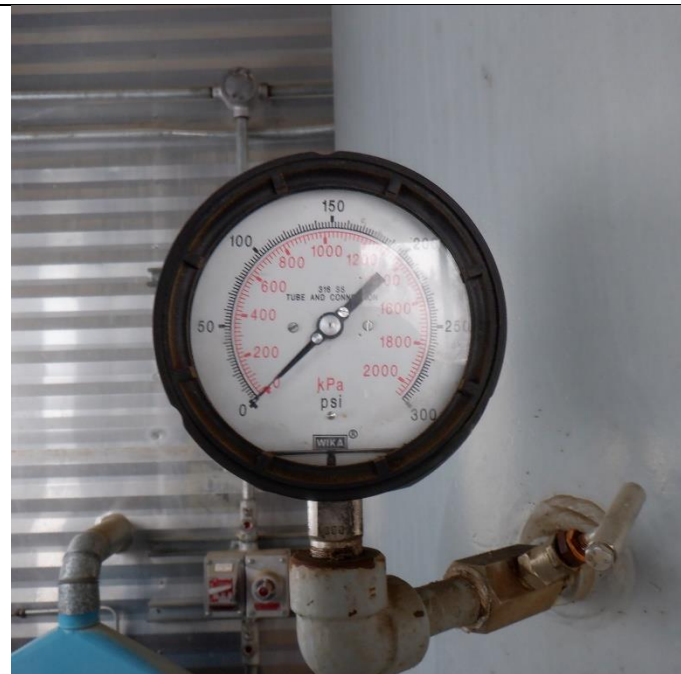
PI overview (gauge oil drained out).
