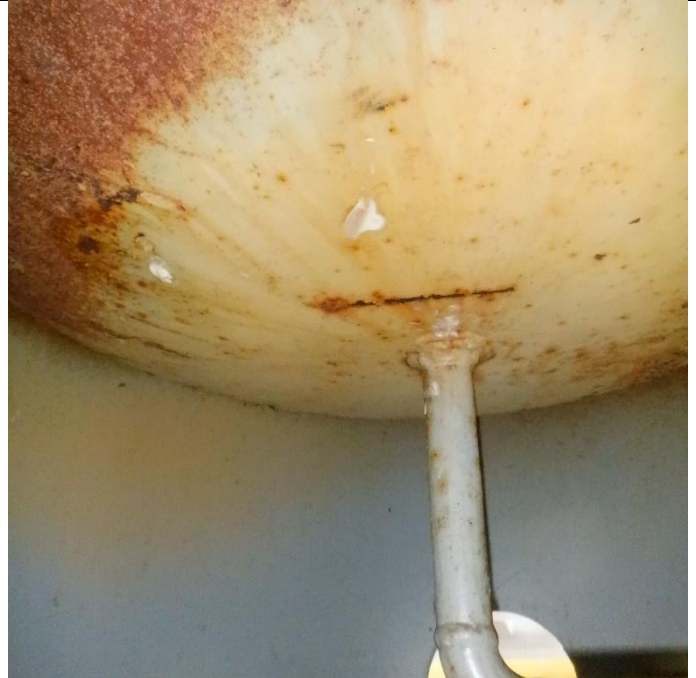
Bottom head of vessel (paint deterioration).
